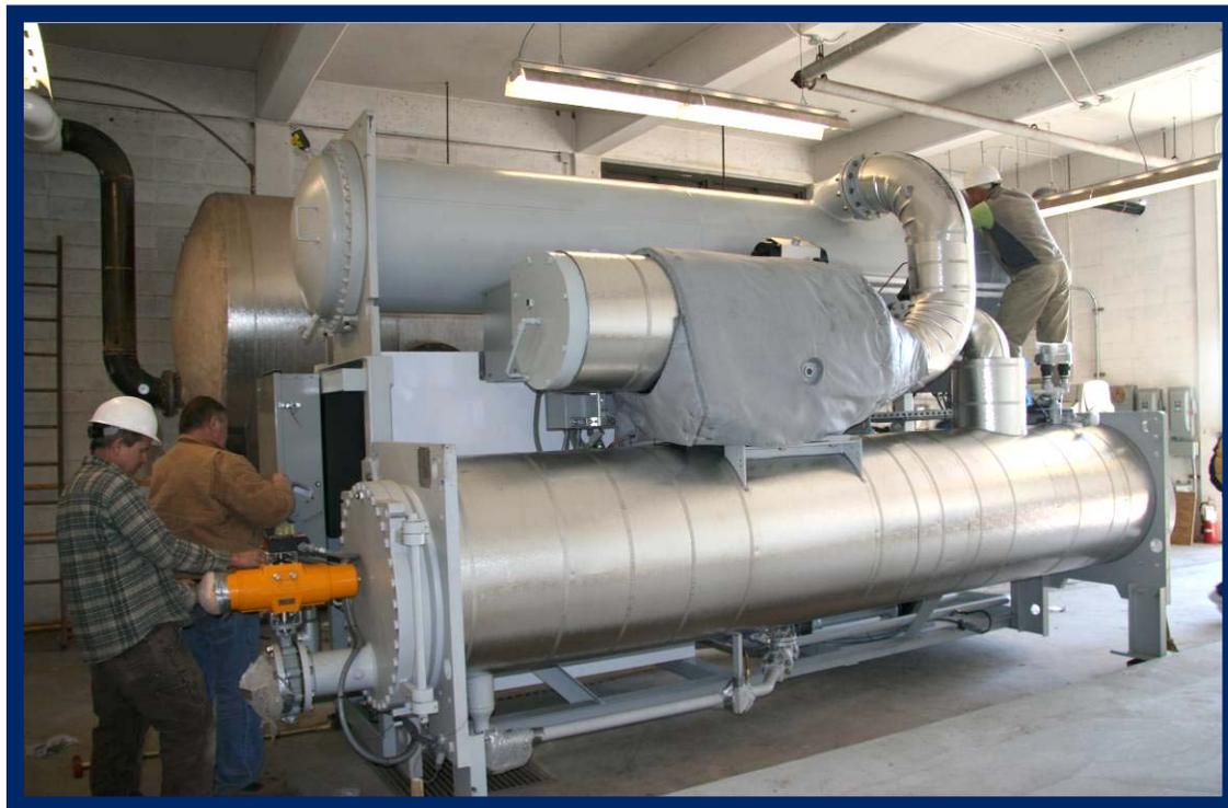
Photo: Workers install a Pratt and Whitney Power Systems 280 kW PureCycle geothermal unit at the Oregon Institute of Technology.
